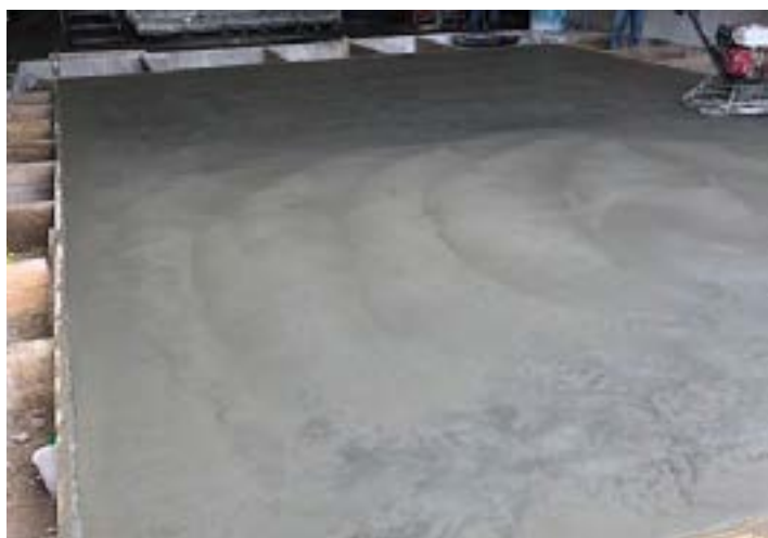
Foundation prepped for boring mill install
